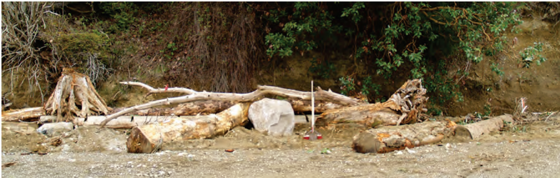
Fig. 1. LWD anchored by auger, chain, and stones, with vegetated upland buffer: a viable alternative to bulkheads. Under construction, above, and completed project, below, during a 17.5 ft tide. Eld Inlet, Thurston Co.
