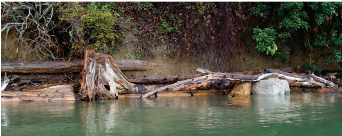
Fig. 1. LWD anchored by auger, chain, and stones, with vegetated upland buffer: a viable alternative to bulkheads. Under construction, above, and completed project, below, during a 17.5 ft tide. Eld Inlet, Thurston Co.
